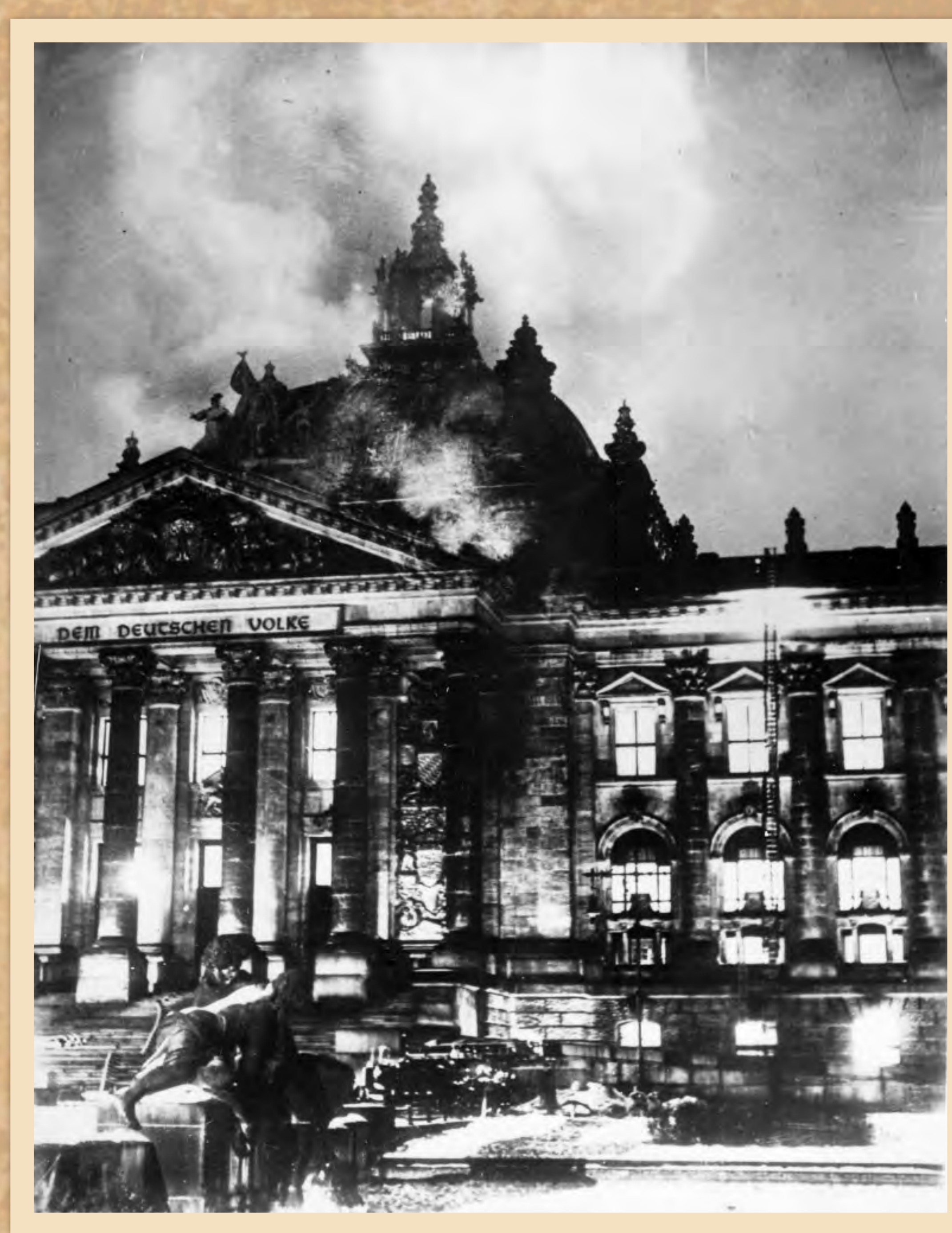
Reichstag fire, February 1933. Photo from National Archives and Records Administration
